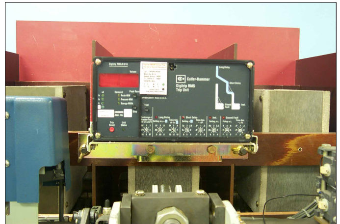
Fig. 48 Overview: Trip Unit Installed on the Breaker.
