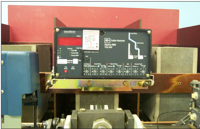
Fig. 54 Trip Unit Assembly Mounted on the Breaker.
