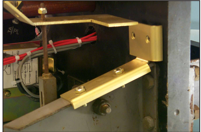
Fig. 43 DTA Mounting Bracket Installed on the Right Breaker Foot.
