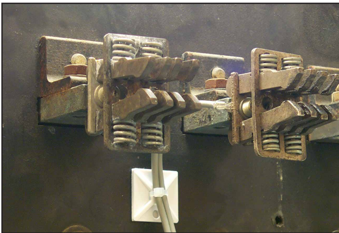
Fig. 36 HV Wires Connected to the Top Breaker Stabs.
