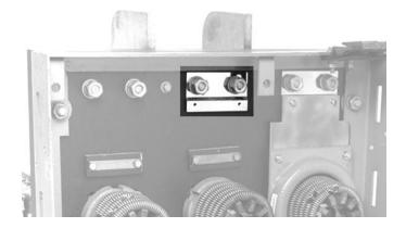
C. Remove and discard the six bolts and washers (one row) located directly below each top Finger Cluster.
