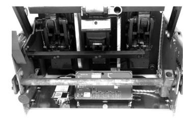
F. Route the External Harness towards the right side of the Breaker, then up towards the DTA Assembly. Remove the top front screw securing the DTA mounting bracket. Using the two wire clamps and the screws provided, secure the External Harness to the DTA.
