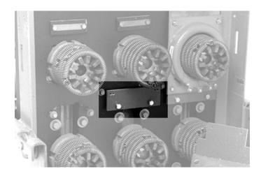
NOTE: Because of the physical differences between the Version "S" and "T" Breakers, different numbers of spacers are used for top and bottom Sensor Assembly mounting, as well as different screw lengths. See the following table and notes for specifics. Page 5
