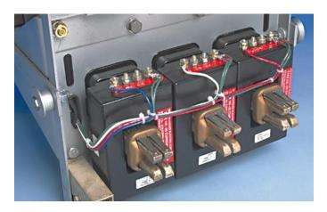
A. Slide a Sensor over each bottom Breaker Stab. The terminals of the Sensors should face upwards.
