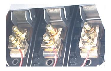
A. Route the PT Wires between the left Trip Unit Assembly Mounting Bracket and the left Arc Chute. Continue by routing the PT Wires down into the Breaker towards the Copper Connectors installed in Step 3.
