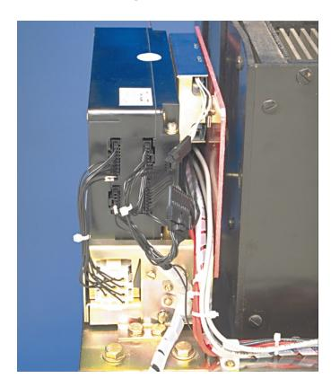
A. Feed the Sensor Harness through the hole in the left side of the Aux. CT Module. Connect the Sensor Harness to the proper terminals on the Aux. CT Module. Refer to Section 12 of the Retrofit Application Data, supplied with the Retrofit Kit, for detailed wiring specifications.
