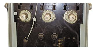
J. Optional HV Wire Routing. If the opening in the Breaker Back Plate does not exist, or if another Breaker Component is blocking the opening, the HV Wires can be routed to the right side of the Breaker then over the top of the Breaker Back Plate.
