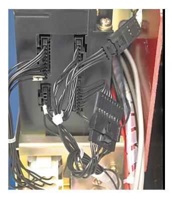
M. Use the wire ties, wire clamps, and self adhesive wire clips provided to dress all wires and harnesses to keep them away from any moving parts within the Breaker. NOTE: The self adhesive wire clips should be attached to the right Breaker side panel to secure the Sensor Harness. The wire clamps should be attached to the hardware mounting the Aux. CT Module and the Trip Unit, as shown, to secure the Sensor Harness, External Harness, and PT Extension Harness.
