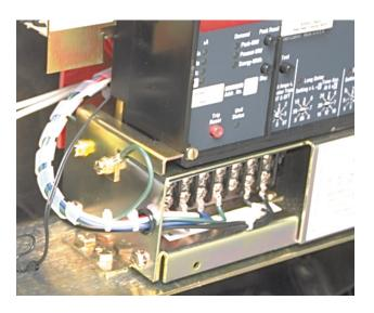
G. Route the DTA Extension Harness between the Glass Poly Insulation Barrier and the back of the Trip Unit, then down along the back edge of the right Trip Unit Support Bracket and into the Breaker to the DTA Assembly. Connect the wire from the DTA Extension Harness marked with "+" to the terminal to which the "+" DTA Wire is attached and the unmarked wire to the other terminal.
