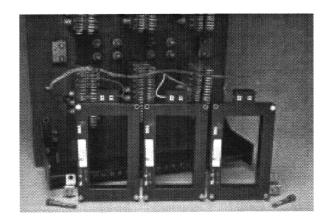
G. Remove the top bolts securing the Secondary Contact Rack near the bottom of the Breaker. Mount the Sensor Assembly to the Breaker Frame, as shown, using the hardware.
