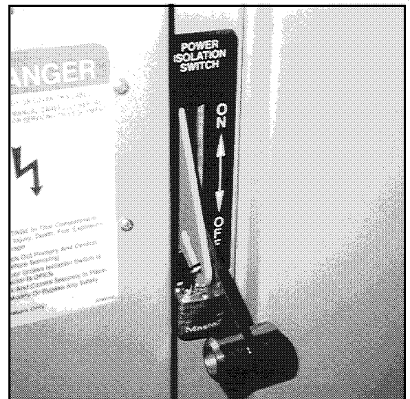
Fig. 9 Isolation Switch Lockout
