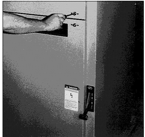
Fig. 46 Preparing For Initial Energization
