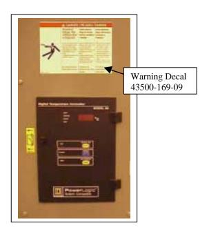
Photo 6. Model 98 Decal Installation
